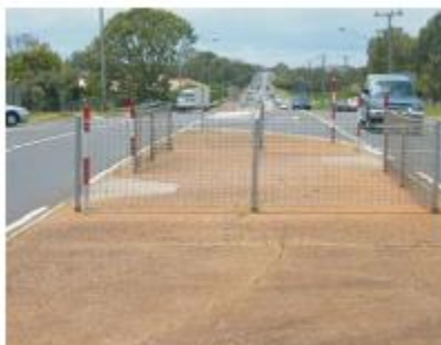
Figure 2.10 – Pedestrian fencing on a median
